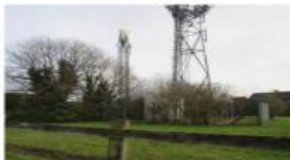
Figure 7: View of telecommunications mast and reservoir north of Parcel B.
